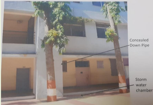
DOWN PIPE TO CHAMBER
